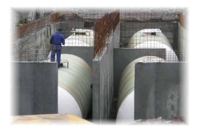
The tanl will be covered with the same type of gravel specified above until it covers 70% of its total volume of the tank.
